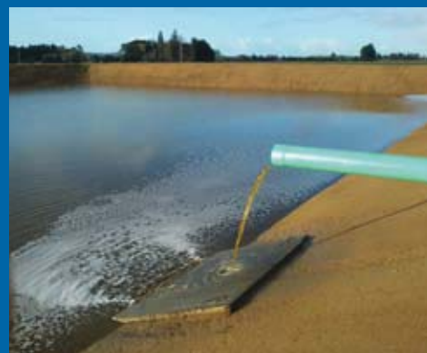
New effluent pond at Shenstone
