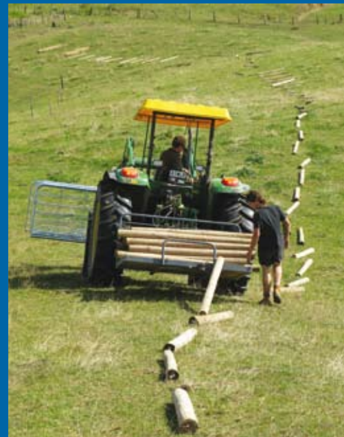
Laying a new fenceline at Annandale
